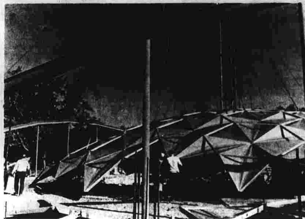
Dome to protect tracks
